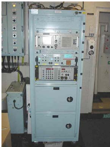
19" equipment rack, housing two lockable cabinets.
